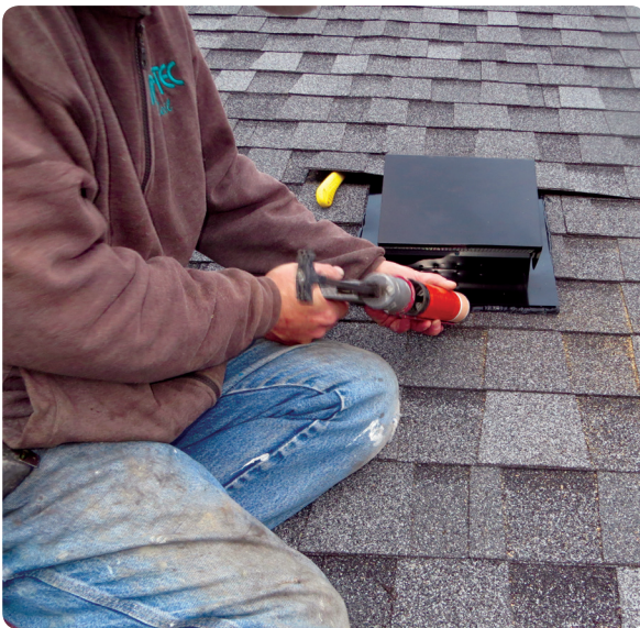
Bathroom and kitchen vents should be vented through the roof — not into the attic.
