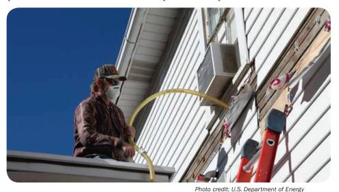
Existing above-ground sidewalls are most commonly insulated by removing siding or drilling holes into the sidewall and blowing loose-fill insulation into cavities.
