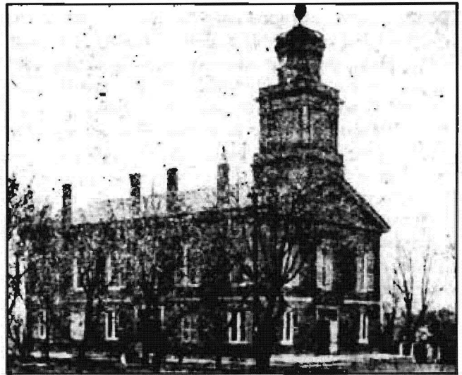
Fig. 1. Marion County Courthouse, 1853-1900. Architect: Charles Levis (From: Palmyra Spectator , July 19, 1900)
