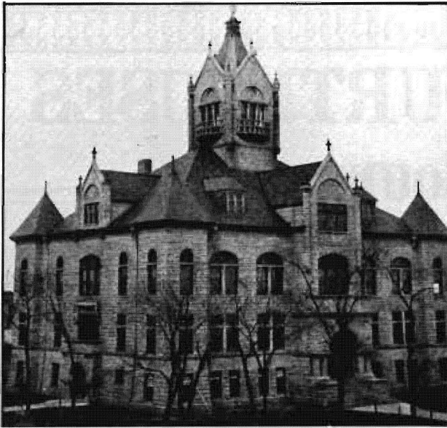
Fig. 2. Adair County Courthouse, 1897-. Architect: Robert G. Kirsch. (Courtesy: State Historical Society of Missouri)
