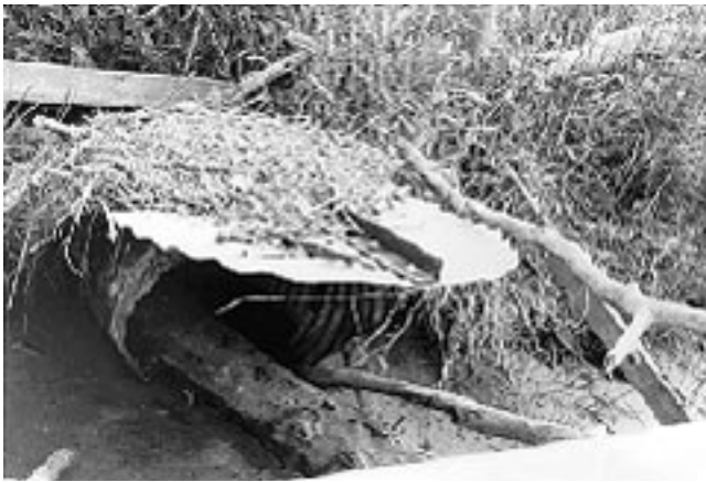
Figure 7. Remove debris from the pipe spillway inlet area.
