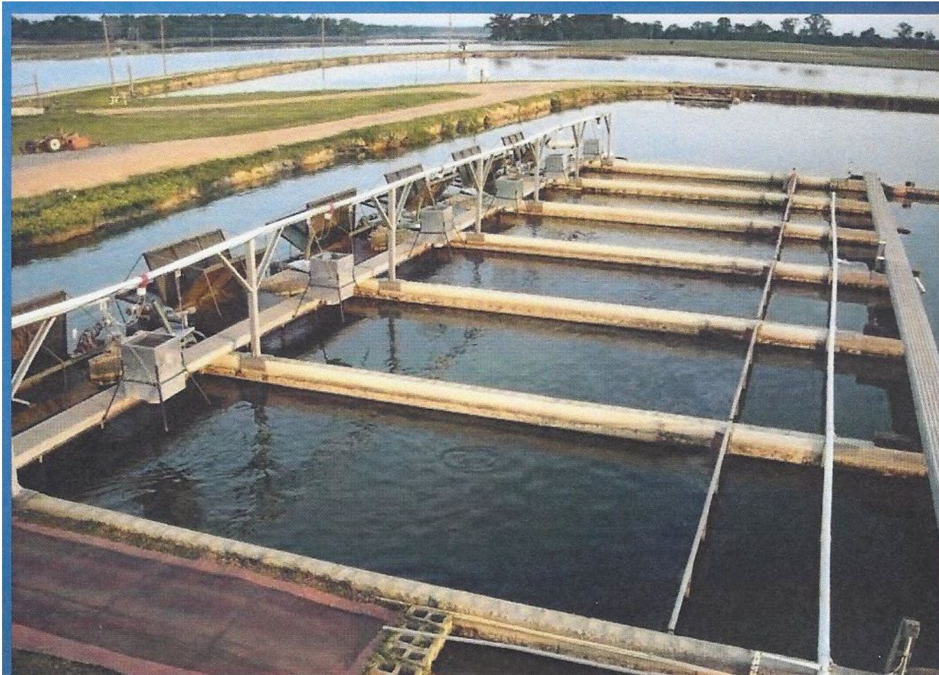
Auburn In-pond Fixed Raceway
