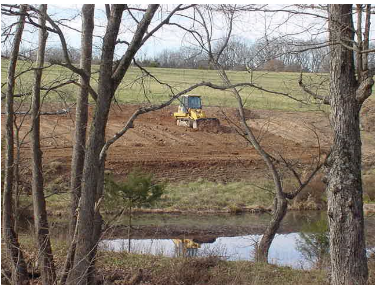
Site Preparation in Morgan County, Missouri; 0.28 Acres; Cost = $3,500
