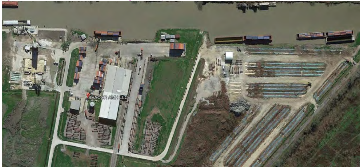
Figure 42. Seacor AMH container-on-barge (COB) operation at Port Allen, LA (Jan, 2019)
